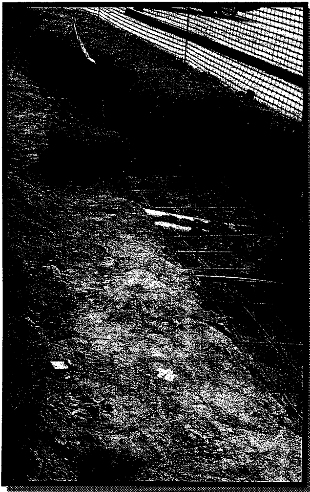
Chesterfield County Veterans Memorial Wall FOOTING POURED JULY 20, 2000 Photo by: W. Baxter Perkinson, Sr. (TOBAC)
